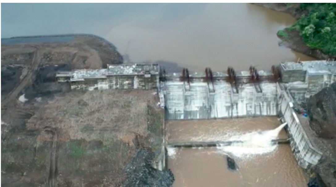
Figure 2-24 : Discharge of water through a sluice valve
