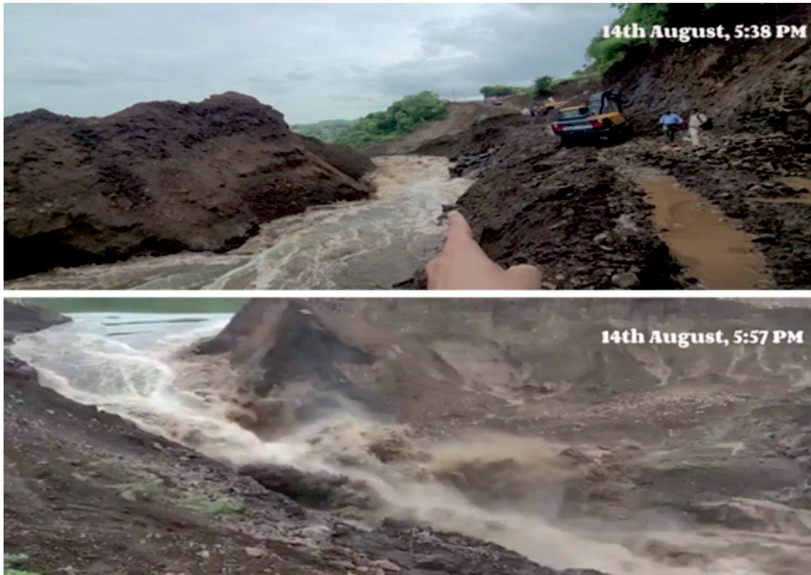
Figure 2-29 : The breach in the dam embankment
