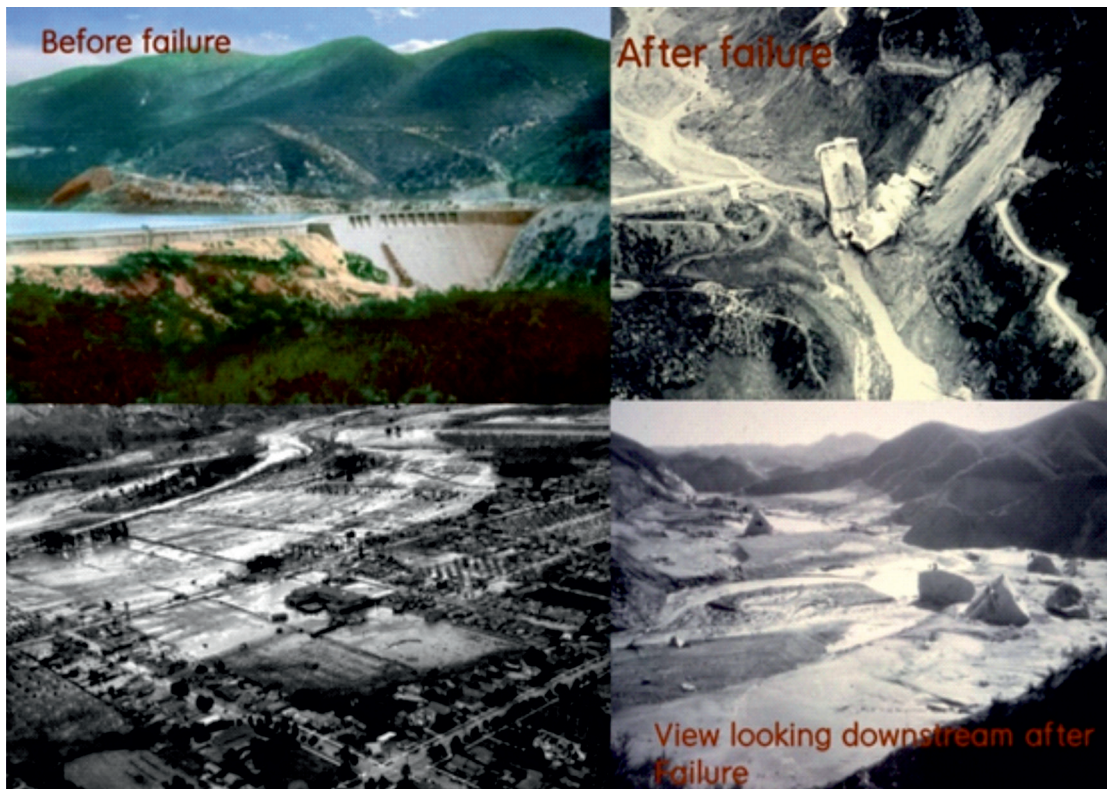
Figure 1-6 : Losses due to failure St. Francis Dam (California, 1928) Source: J. David Rogers, 2013 AEG Shlemon Specialty Conference
