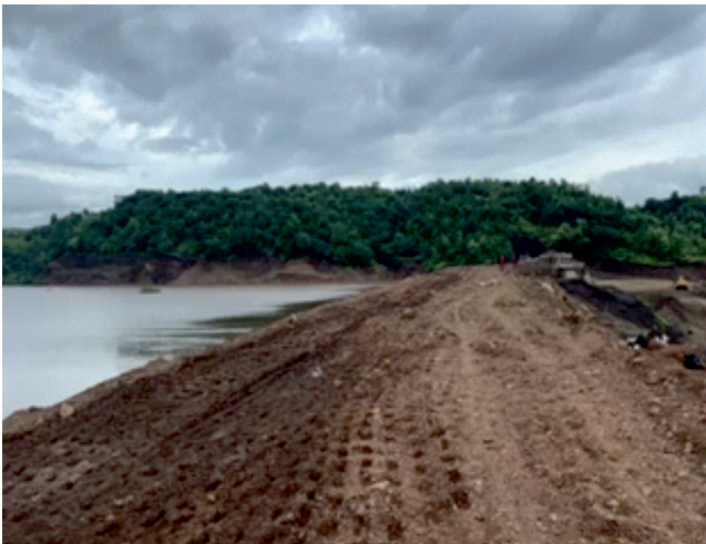
Figure 2-2 : Roller compaction of Embankment crest
