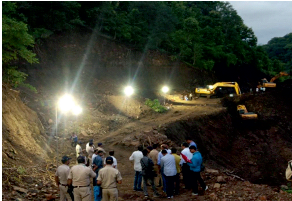
Figure 2-10 : Excavation on right flank to make a channel
