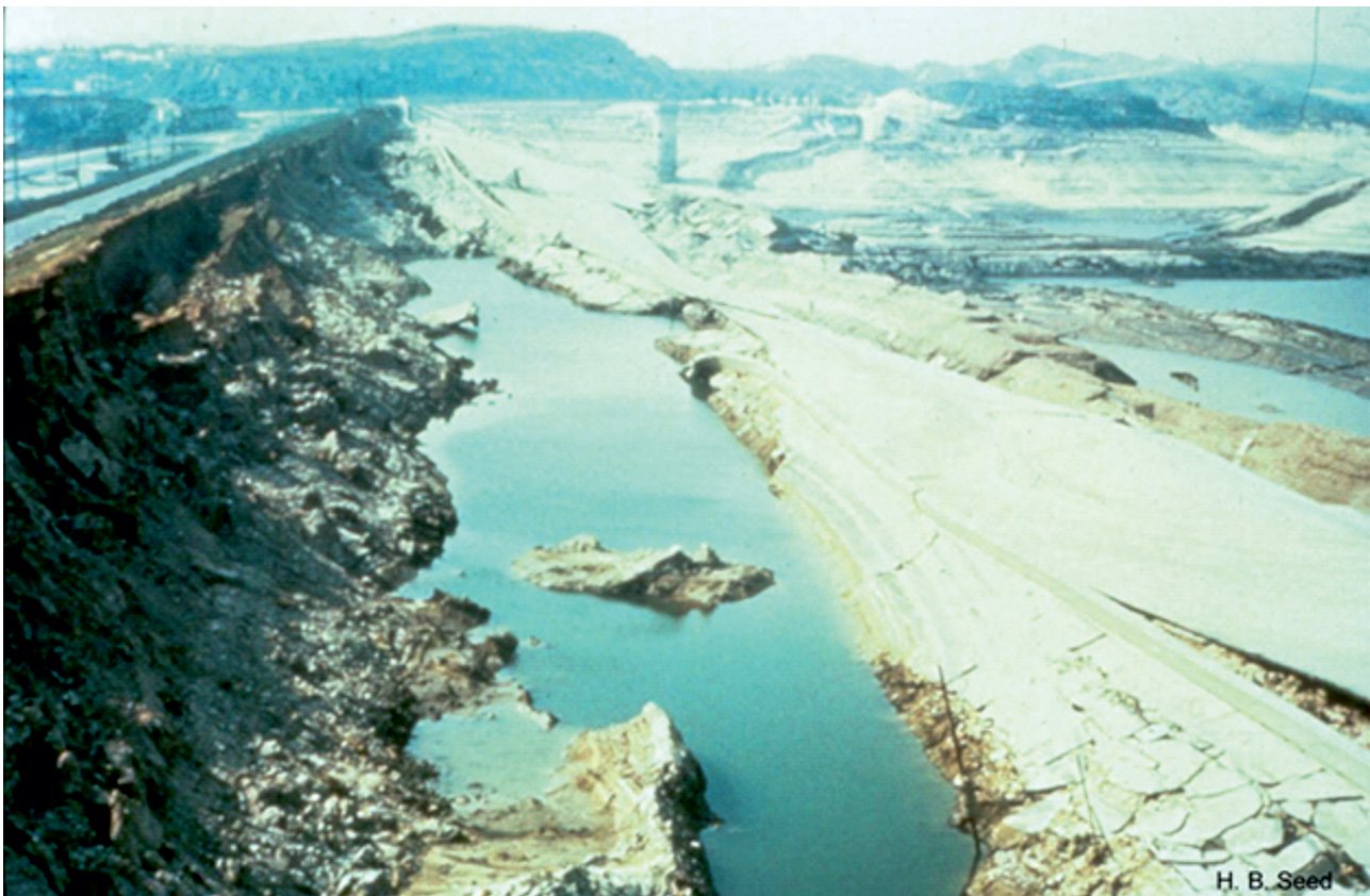
Figure 1-9 : Upstream slope of the dam after earthquake and draining of lake; Tower No. 2 is in the background (standing).
