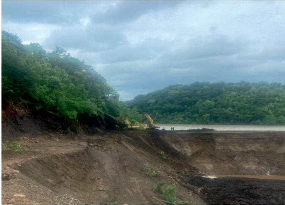
Figure 2-9 : Excavation for bypass channel
