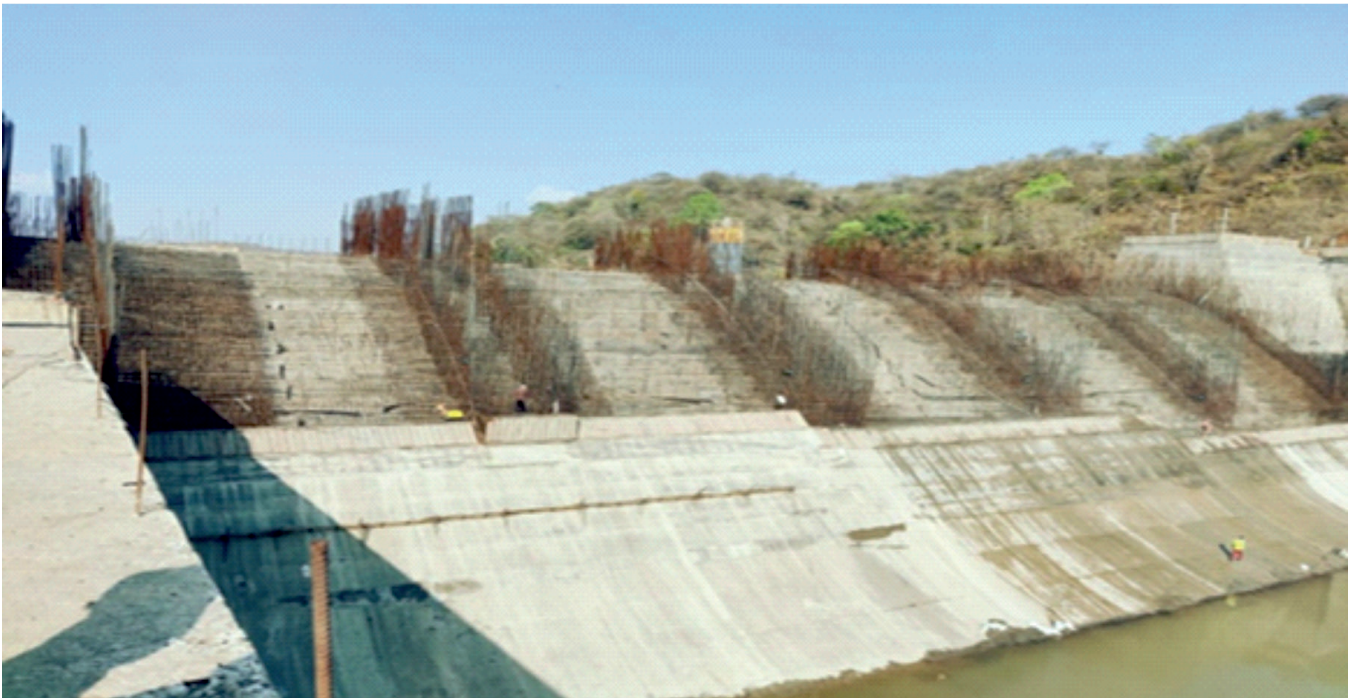
Figure 1-20 : Spill way under construction
