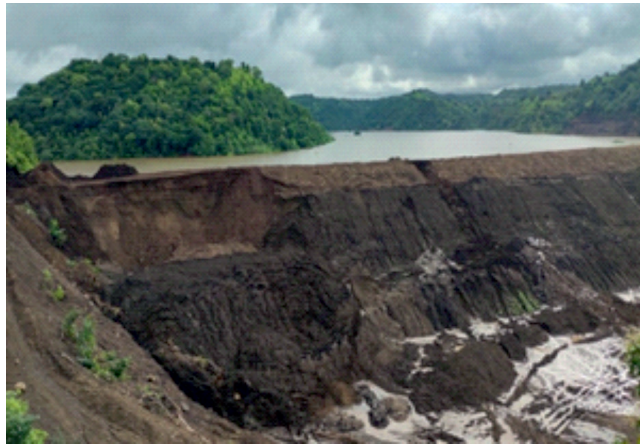
Figure 2-4 : Slacking of soil from the embankment
