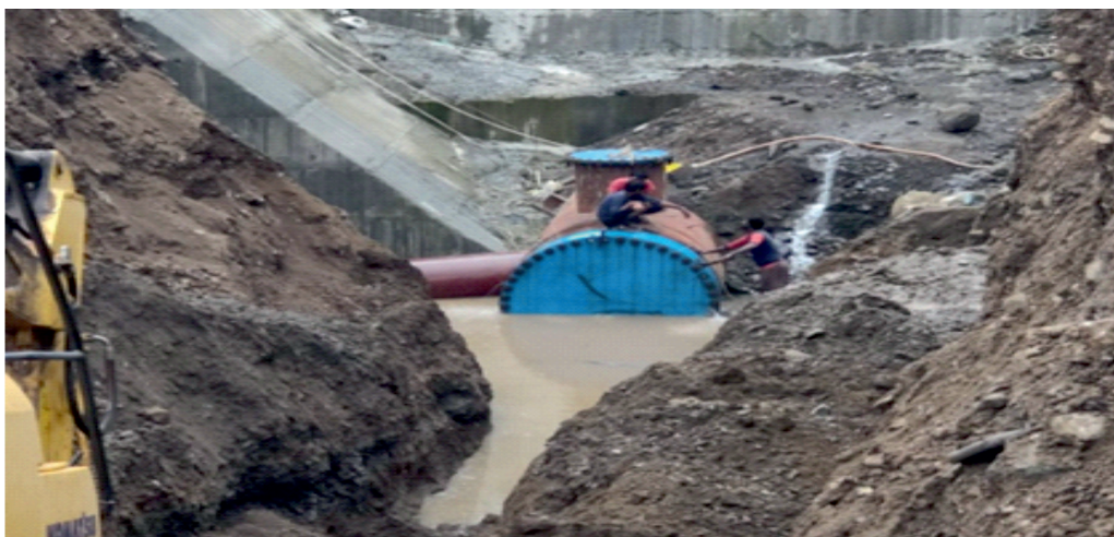
Figure 2-6 : Efforts to open the Sluice gate which was closed
